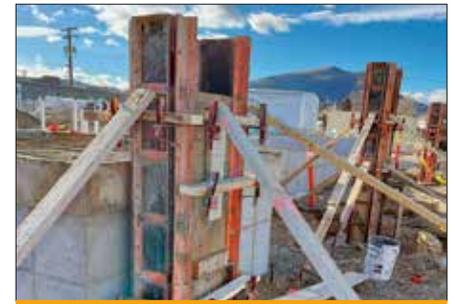
At the end of October, Dick Anderson Construction and local contractors began site preparation. It has been a very productive few months of moving and leveling dirt, burying pipe to connect to city water and sewer, installing the stormwater detention system, and completing concrete work for footings and the foundation.
