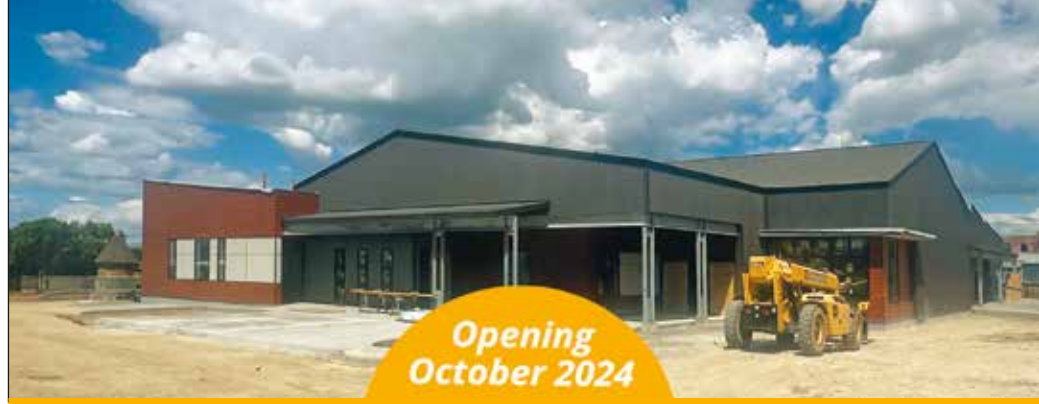
Community Food Resource Center under construction, July 2024.
